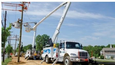
Figure 1: Use of Bucket truck for Electrical System Maintenance [2]
