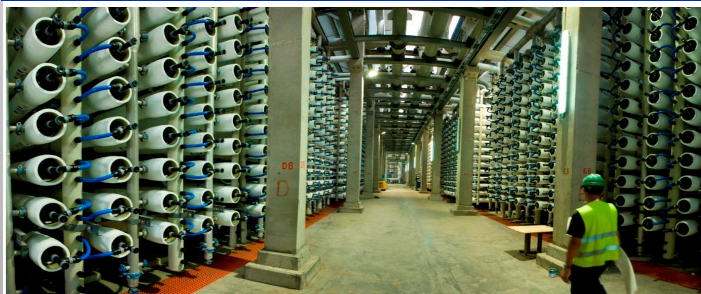
Reverse Osmosis Membrane System in IDE Hadera Plant.
